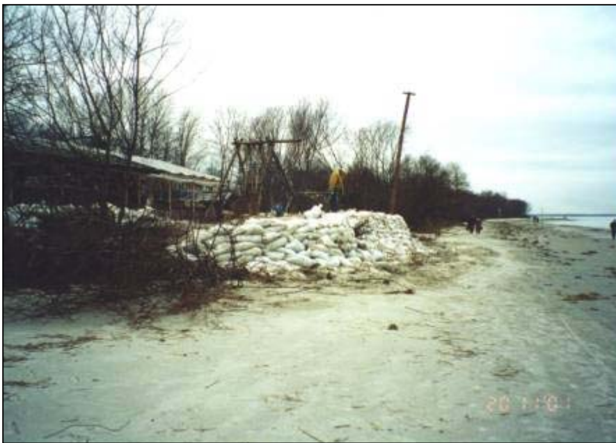
Fig. 8: Temporary defence measures in the place of the washed-off foredune. Jurmala, November 2001. Photo: G. Eberhards, November 2001.
