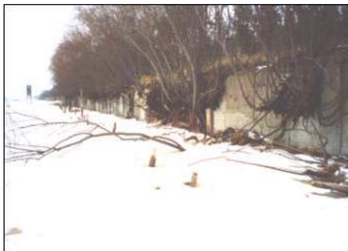
Fig. 7: The concrete base of the foredune, erected after the storm of 1969 and exposed again after the erasure of the foredune in November 2001. Photo: G. Eberhards, November 2001.
