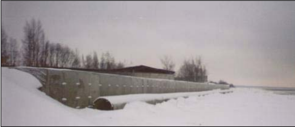
Fig. 10: The revetment of Daugavgriva exposed after the storm of November 2001. Photo: R. Povilanskas, December 2002.
