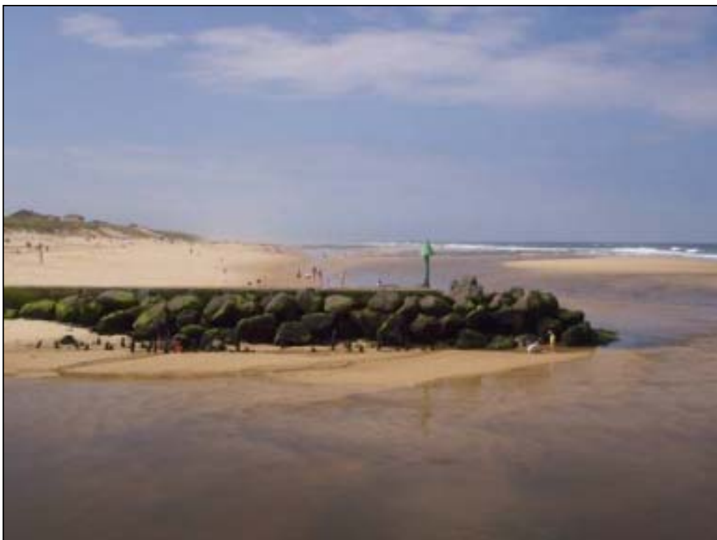
Fig. 9: Hard structures – groins.
