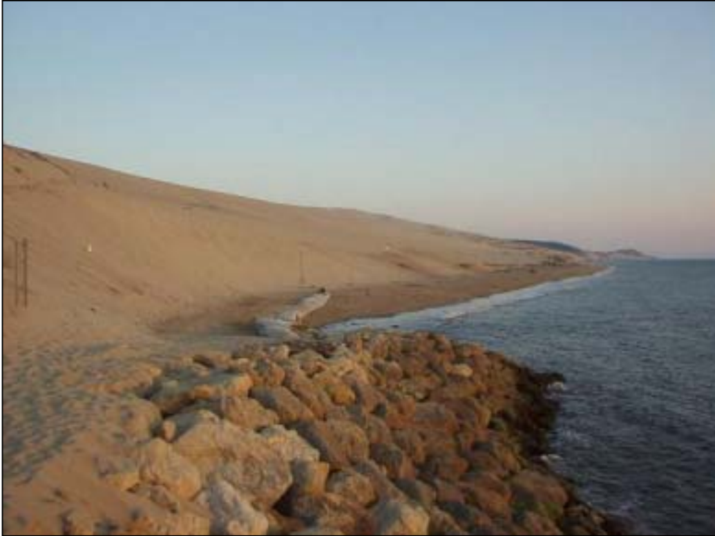
Fig. 10: Hard structures – rock revetments.
