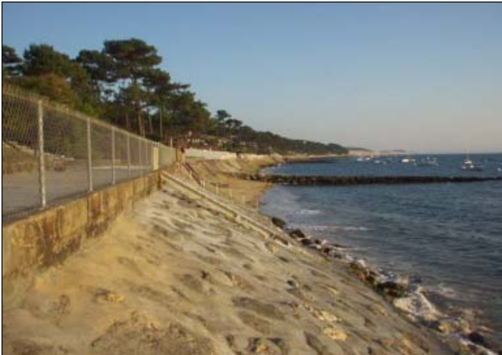
Fig. 8: Hard structures – seawall.
