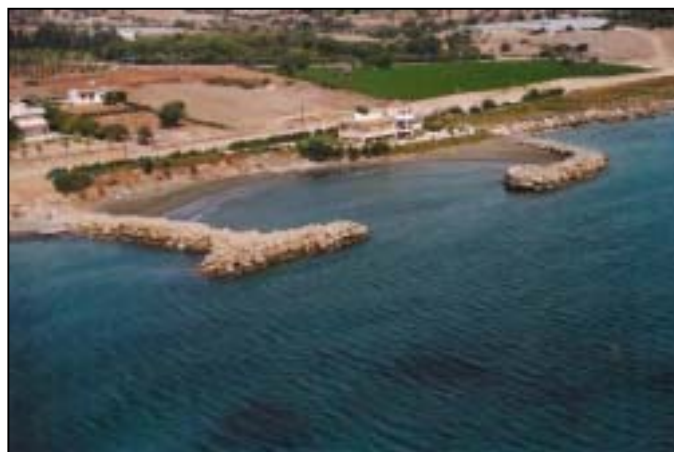
Fig. 6: Groins illegally constructed to protect private property (Agios Teodoros).
