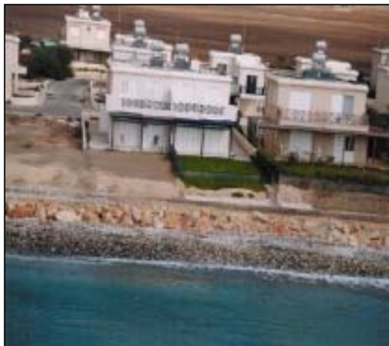
Fig. 3 & 4: Private properties under risk of destruction due to severe erosion. The owners constructed the sea defences illegally (rocky revetments and wooden pile revetments).
