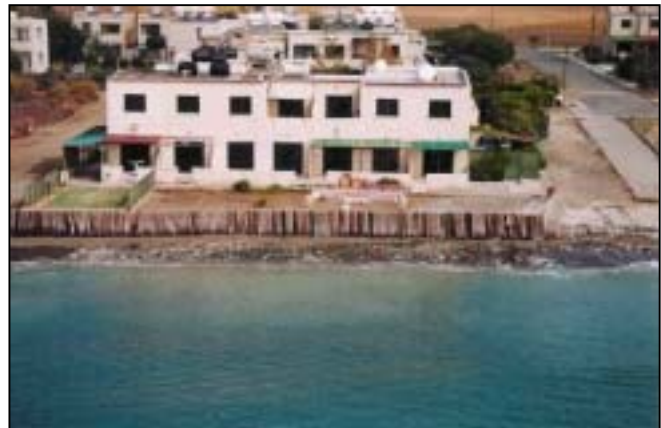
Fig. 3 & 4: Private properties under risk of destruction due to severe erosion. The owners constructed the sea defences illegally (rocky revetments and wooden pile revetments).
