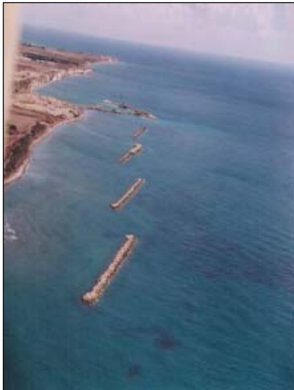
Fig. 10: Offshore breakwaters in Alaminos – view East.
