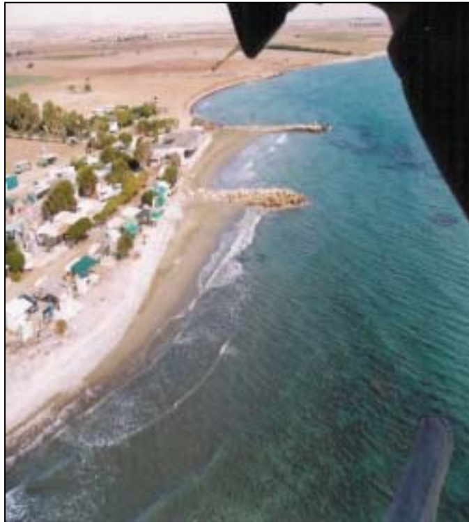
Fig. 7: Groins illegally constructed in Mazotos.
