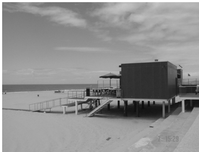
Fig. 3 The new beach's bars aims to fulfil some quality criteria in terms of public services and environmental patterns
