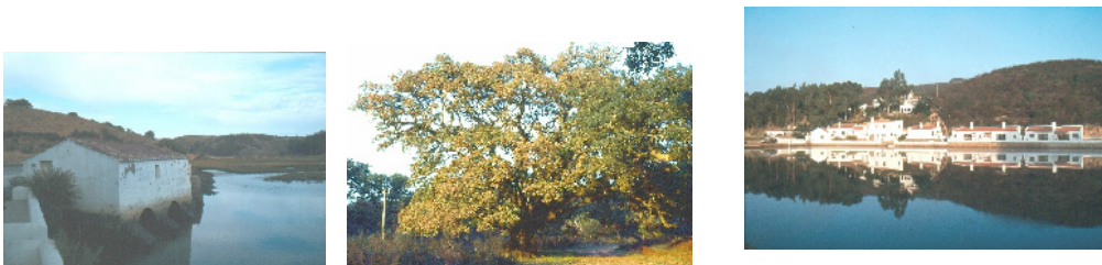
Photo 53-54-55. Water mill in Mira River with the re qualification of the existent buildings
