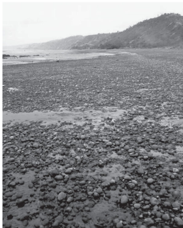
Fig. 4. The same locality as it appears today, after being affected by strong waves during the 1997-1998 El Niño event. The camaroneras were completely destroyed (see some remnants in the background) and the undermined coastal road has remained interrupted at several points.
