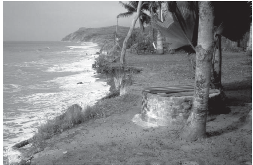
Fig. 8. A water well, dug some tens of metres inland at the time, is now close to the cliff edge.
