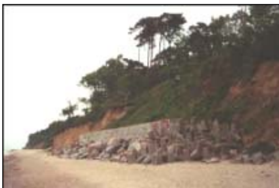
Fig.16: Combined seawall in Rewal (plus tetrapods)
