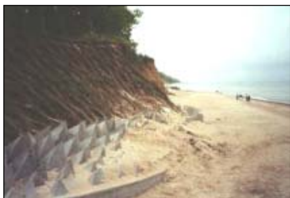
Fig. 19: Combined wood sticks with seawall.
