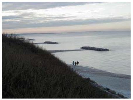
Fig. 11: New breakwaters with the formation of tombolos behind it.
